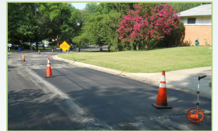
New patch is flush with existing pavement
