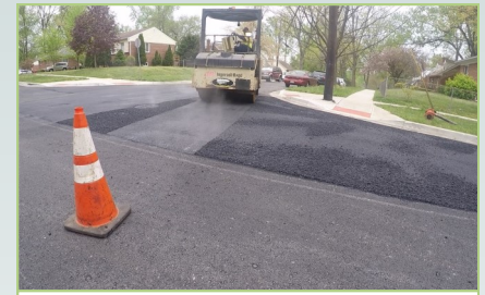
New asphalt is placed and compacted
