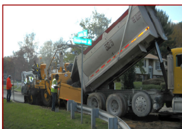
Typical asphalt paving operation.
