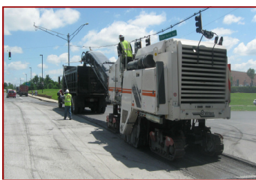
Typical milling operation.
