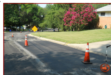
New patch is flush with existing pavement
