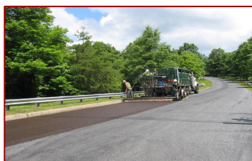
Micro surfacing application
