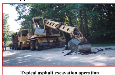
Typical asphalt excavation operation
