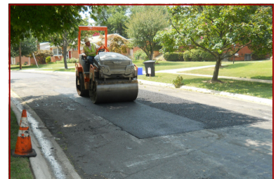
New asphalt is placed and compacted
