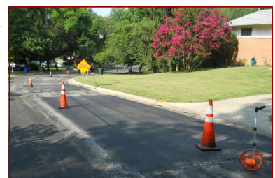
New patch is flush with existing pavement
