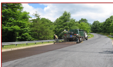
Micro surfacing application
