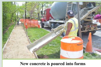
New concrete is poured into forms
