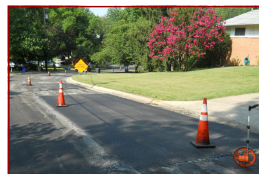
New patch is flush with existing pavement
