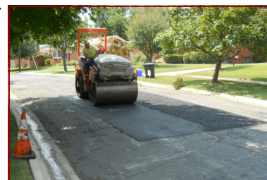
New asphalt is placed and compacted
