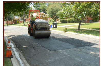
New asphalt is placed and compacted
