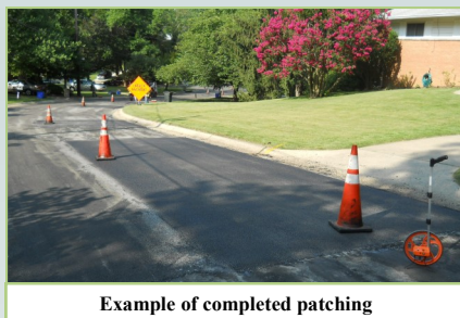
Example of completed patching
