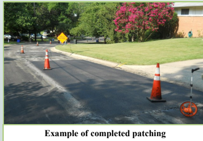
Example of completed patching
