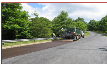
Micro surfacing application
