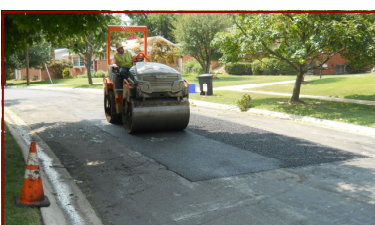
Typical asphalt patch
