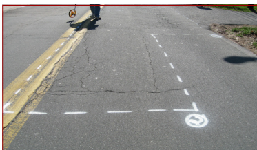
Typical paint markings
