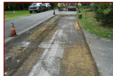
Pavement will be replaced in 2 phases
