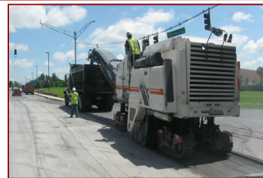
Milling machine excavating
