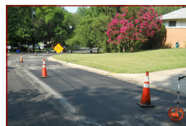
New patch is flush with existing pavement
