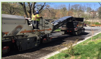
Milling machine patch excavating
