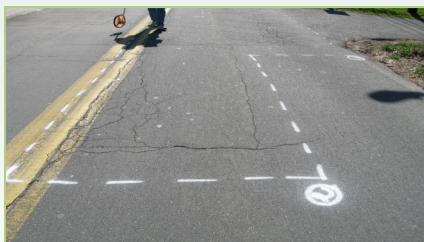
Typical survey paint markings
