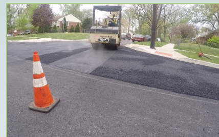
New asphalt is placed and compacted
