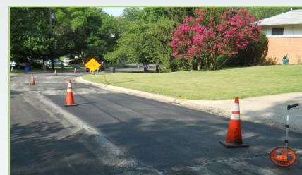
New patch is flush with existing pavement
