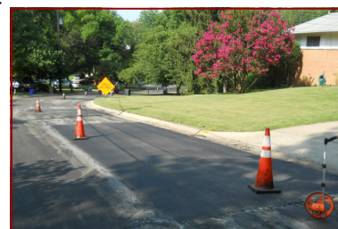
New patch is flush with existing pavement
