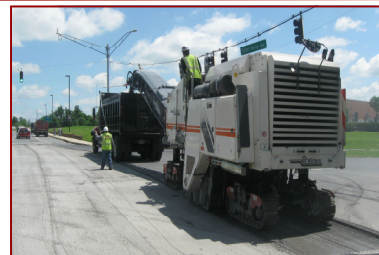
Milling machine excavating
