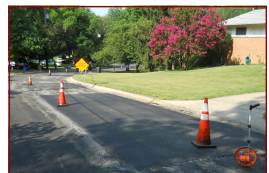
New patch is flush with existing pavement
