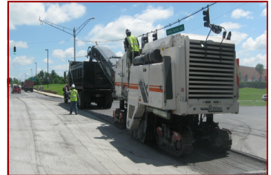
Typical milling operation
