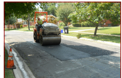
New asphalt is placed and compacted
