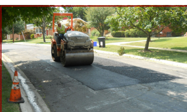
Typical asphalt patch
