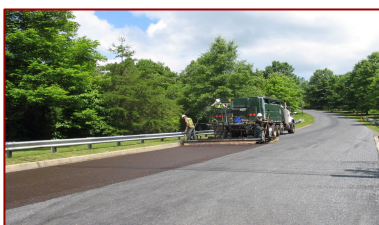
Micro surfacing application
