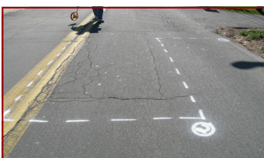
Typical patching paint markings
