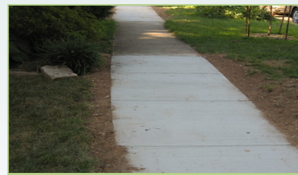
Completed sidewalk repair
