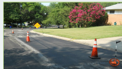
New patch is flush with existing pavement
