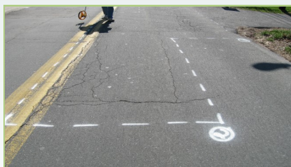
Typical survey paint markings
