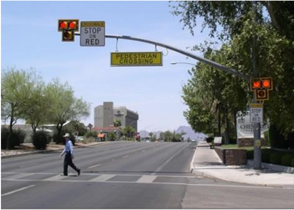
HAWK Signal in Arizona, via Federal Highway Administration
