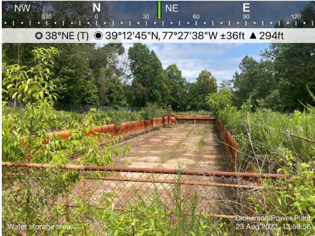
13. View of concrete-lined stormwater management basin (08/23/23).
