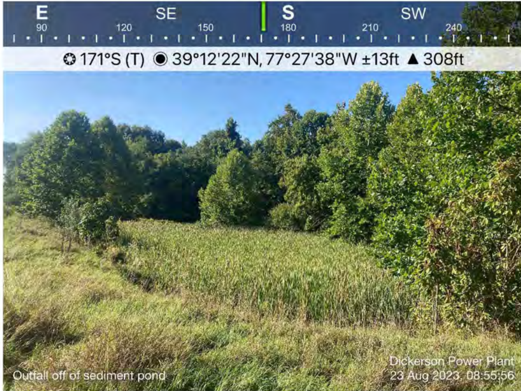
19. View of off-line, man-made stormwater management pond with rip-rap outfall (08/23/23).
