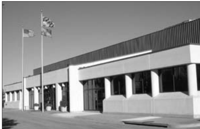
Montgomery County's Recycling Center is state-of-the-art and offers guided tours.
