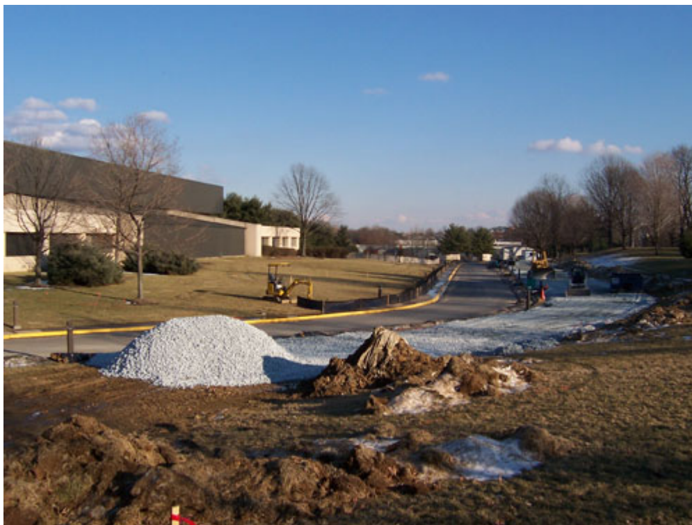
The initiation of work for the Transfer Station improvements
