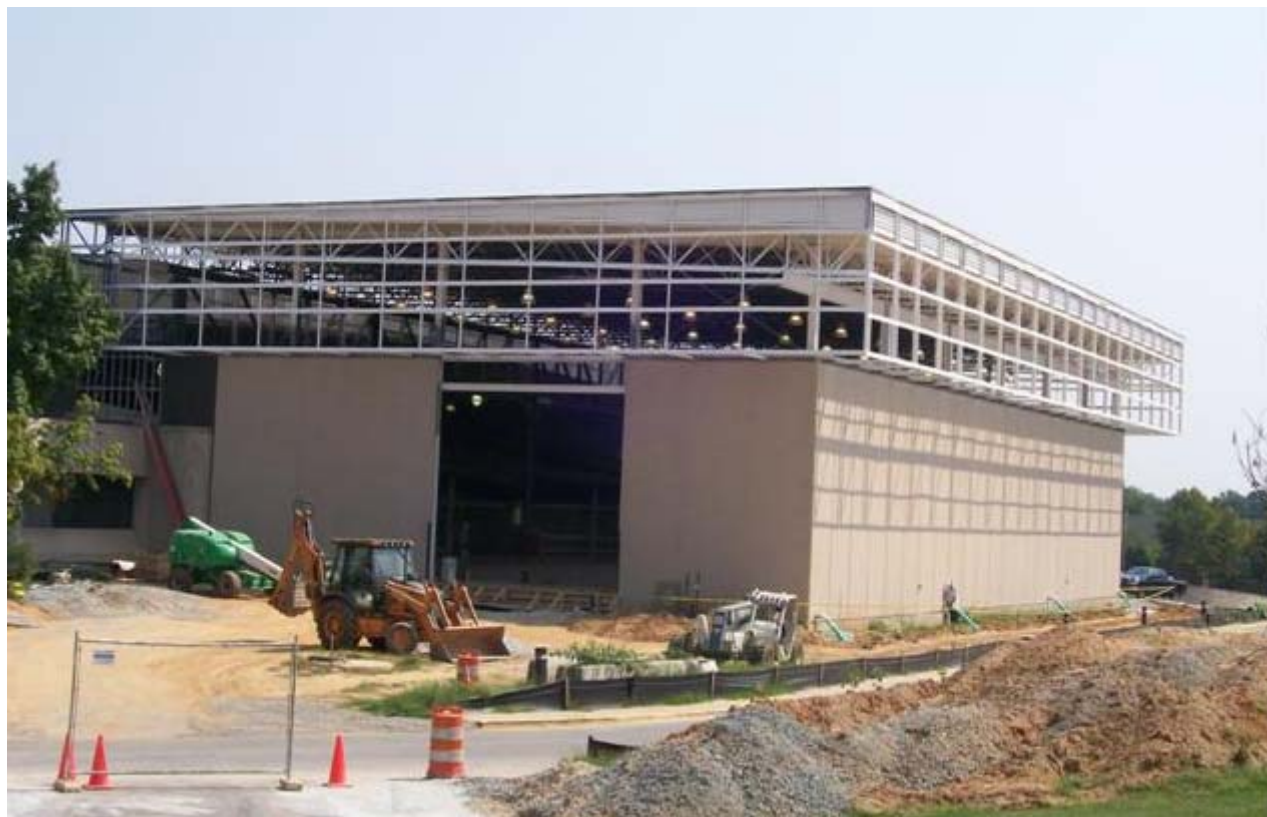
“Construction of the New Transfer Station Building Addition”
