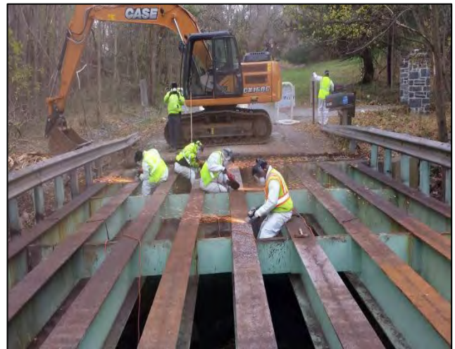
Highway Services Depot Crews replace the bridge deck span along Huntmaster Road in Damascus
