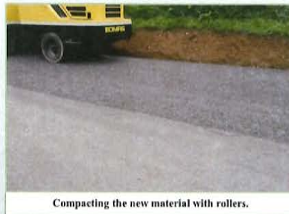
Compacting the new material with rollers.
