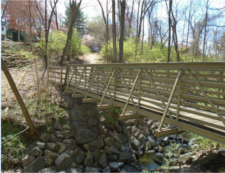
ELEVATION VIEW - TYPICAL PREFABRICATED TRUSS FRP BRIDGE
