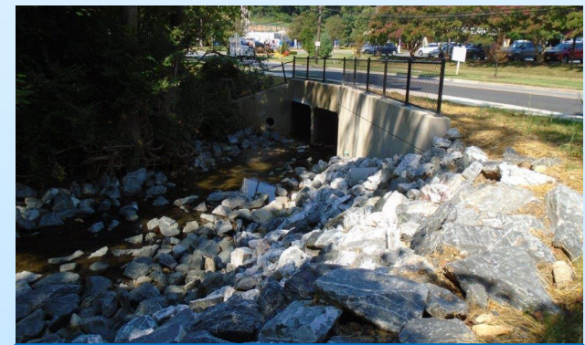
Example of Riprap Slope Protection
