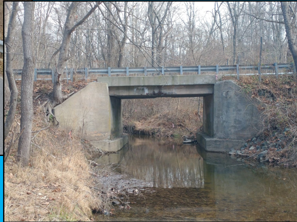
West Elevation (Downstream)
