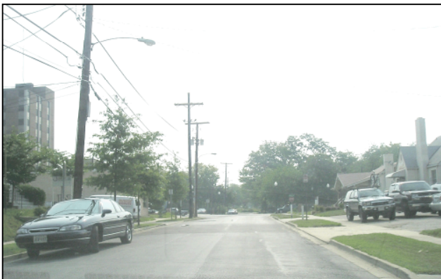
EB Gist Avenue approaching Fenton St.
