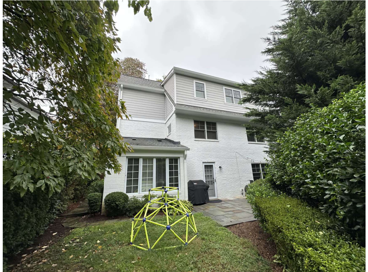
7505 TARRYTOWN ROAD VIEWED FROM REAR YARD TOWARD LEFT REAR FACADE
