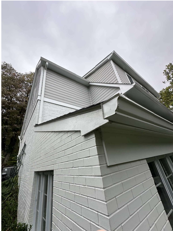
7505 TARRYTOWN ROAD - EXISTING ROOF OVER WALKOUT BASEMENT AREA
