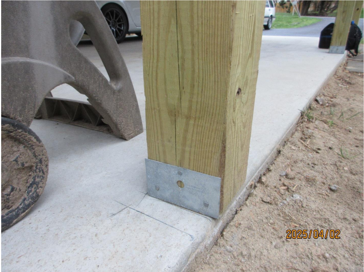
Photo 8: Pre-manufactured post bases are anchored into cast-in-place concrete
