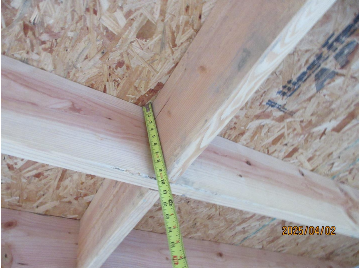
Photo 4: 2x10 Timber Joist with bracing
