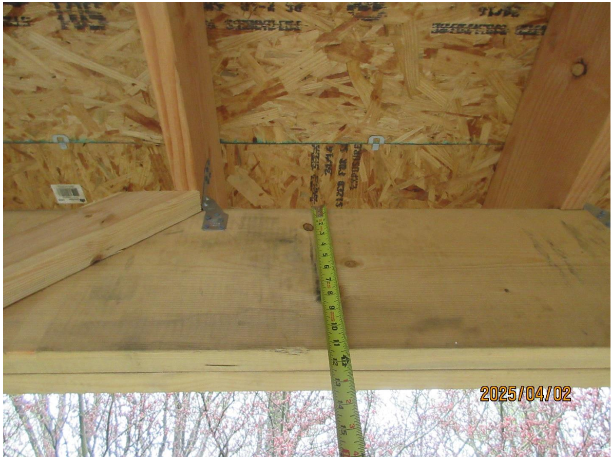
Photo 3: Double 2x12 Timber Beams
