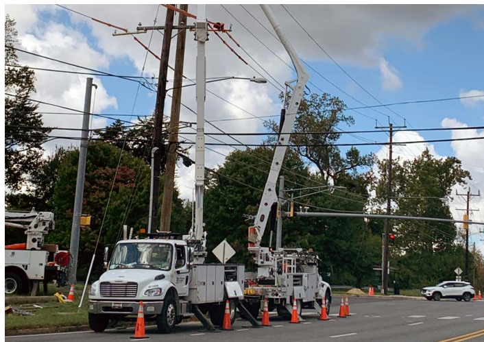
Figure 1. Utility construction for the Veirs Mill Road Flash BRT started on October 2, 2025. Pepco installed three poles to transfer lines at the intersection of VMR and Connecticut Avenue. This relocation is specifically for pedestrian and bicycle safety improvement elements of the project.
