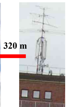
Phone mast Robert-Bosch- Str. 40 Height 30 m, 9 antennas
