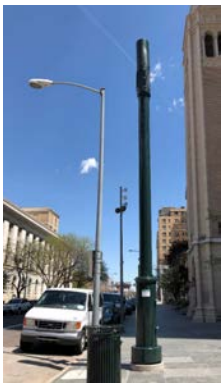
(b) A small cell attached at the top of a streetlight pole (Heilman, 2018).
