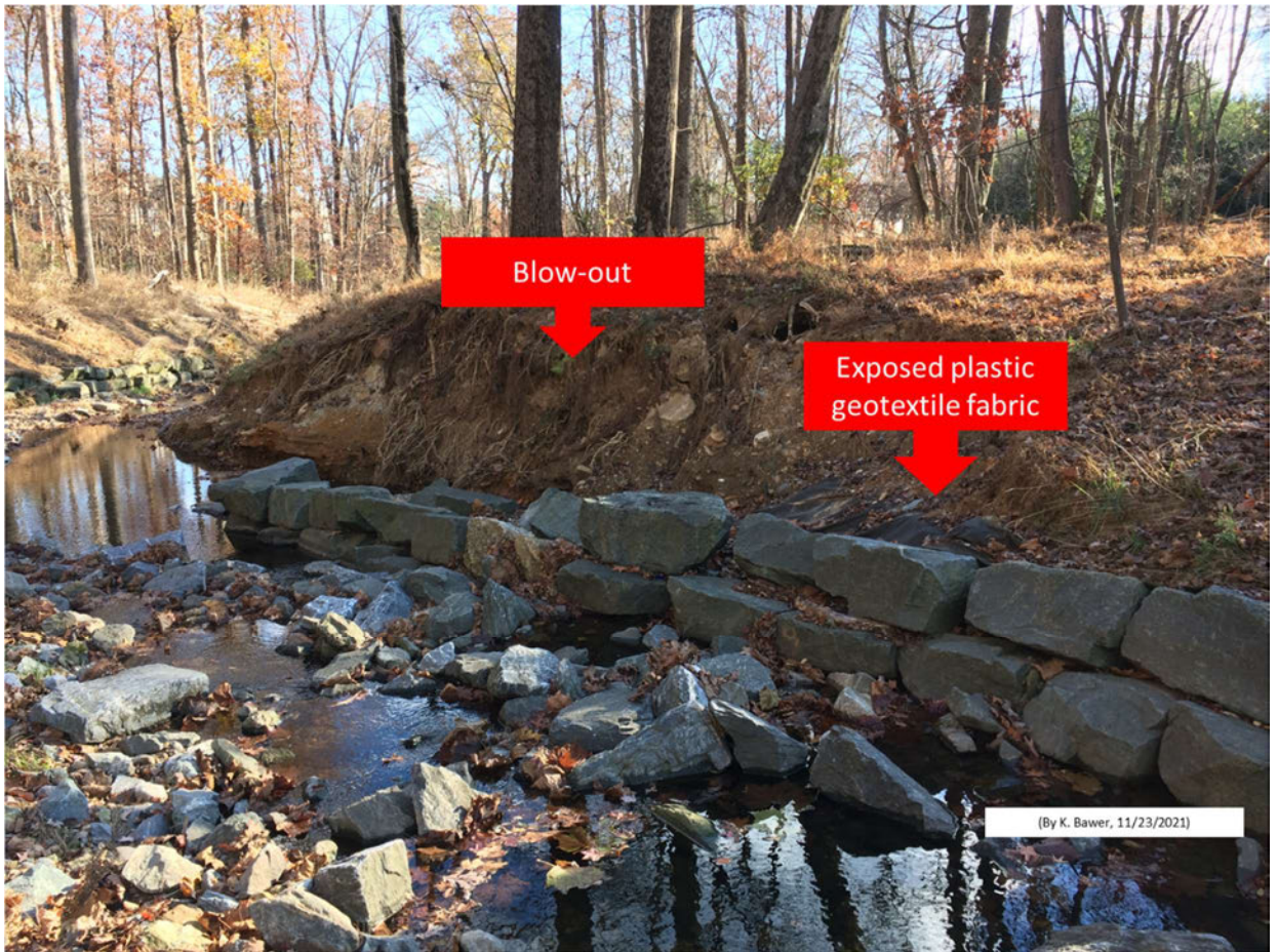
(Above: exposed plastic fabric at Snakeden Branch, Potomac)
