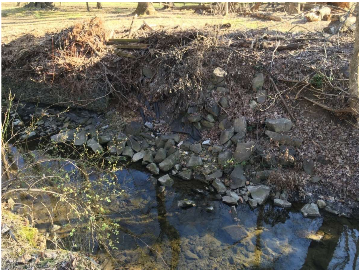
(Above: along an adjacent private property, a failed attempt at stream bank stabilization with Gabion baskets and rip rap along Old Farm Creek Tributary, North Bethesda)
