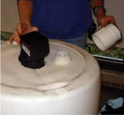
Downspout diverter and overflow adapter (on side)
