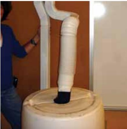
Downspout connection using flexible extender
