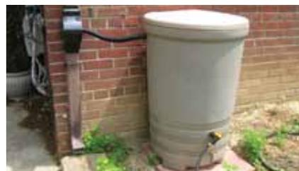
Rain barrel using in-line overflow adapter
