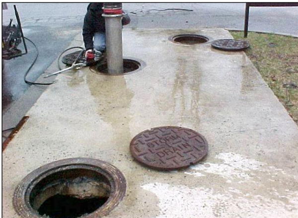
Cleaning an oil grit separator
