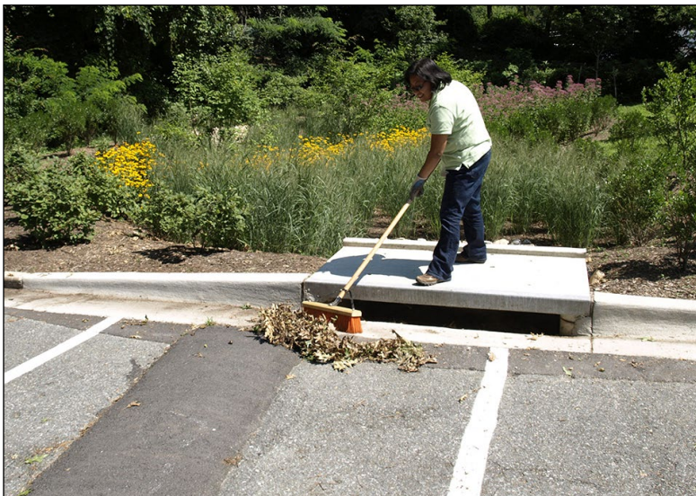
Clear and remove debris from storm drain inlets.
