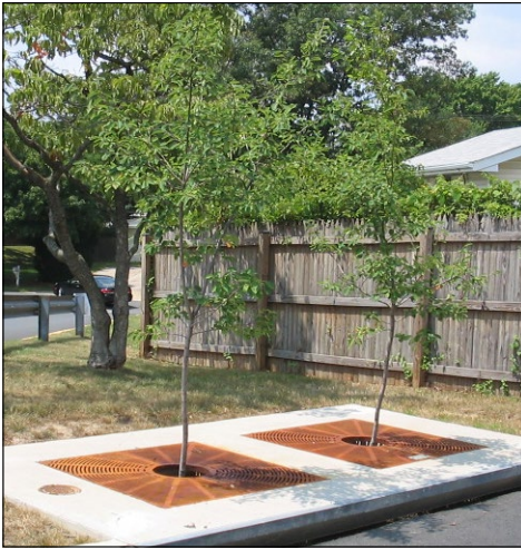
Parking lot with adjacent tree box filters
