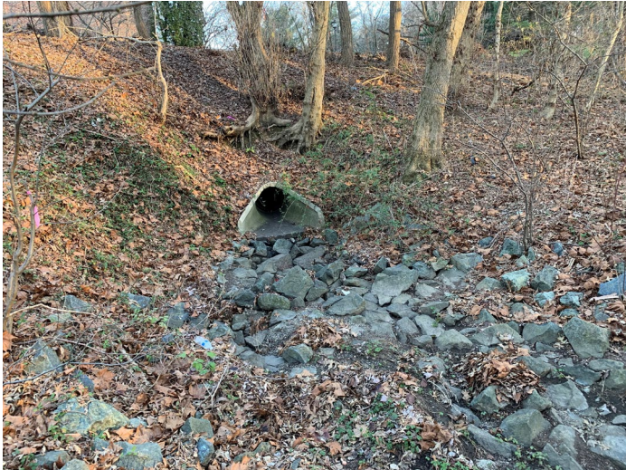
Storm Drain Pipe Outfall
