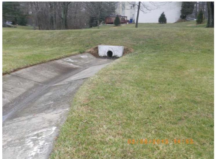
**ABOVE:** Outfalls will be modified by placing riprap and native vegetation around the pipe to minimize the velocity of the water entering the pond.
