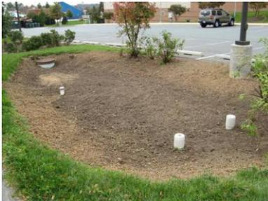
Maintenance crews removed the invasive plants including thistle, mile-a-minute vine, morning glory, pokeweed, milkweed, and others. Crews also repaired areas of erosion, installed riprap at inflow areas to prevent future erosion, replanted the facility, and mulched with double shredded hardwood mulch.
