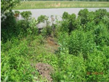
In Fall 2011, DEP completed repair work on three bioretention/biofiltration facilities at Germantown Swim Center. The bioretention facilities were overgrown with invasive weeds.
