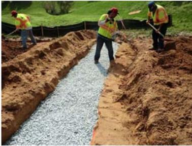
Maintenance crews removed the top 3" of contaminated sand, excavated a 4' wide trench to repair the underdrain and lay filter fabric at the bottom, then back filled with #57 stone, #7 stone, and sand.
