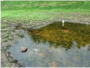
DEP recently completed repair work on the residential sand filter at Sherwood Forest. The filter was clogged, an observation well pipe was broken, and the underdrain pipe was filled with sediment.
