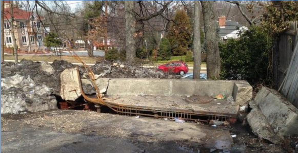
This stormdrain inlet was no match for the snowplow that mangled it. Check all of your structures that may have been exposed to snow equipment. Be sure they are not damaged and are functioning properly.
