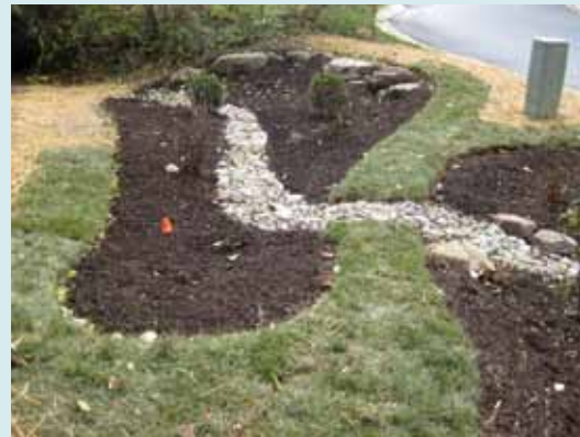
2-celled rain garden just after installation
