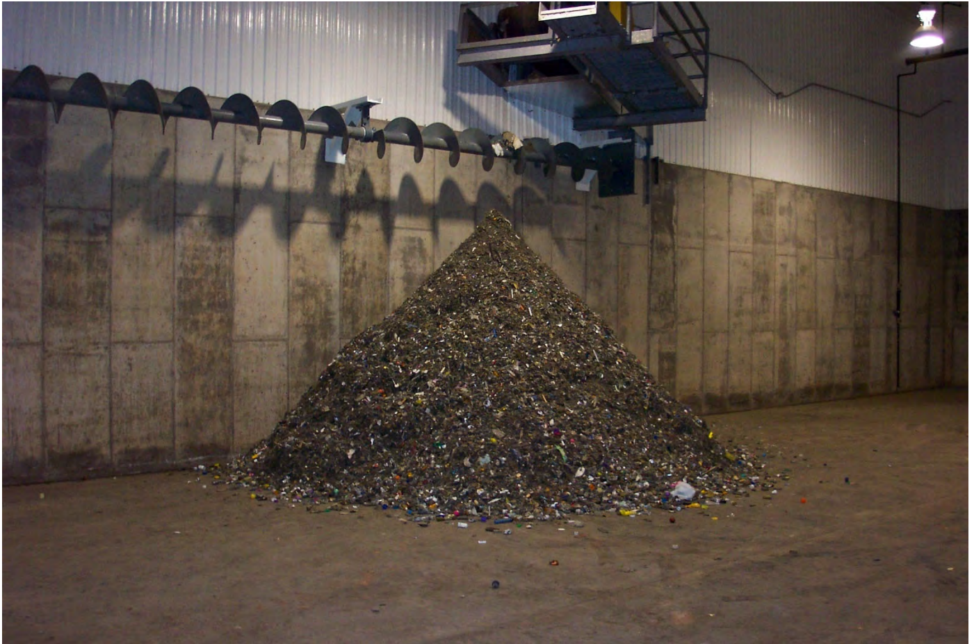
Photo 1 – Co-ground feedstock material belt conveyed to Compost Facility Feedstock Receipt Area
