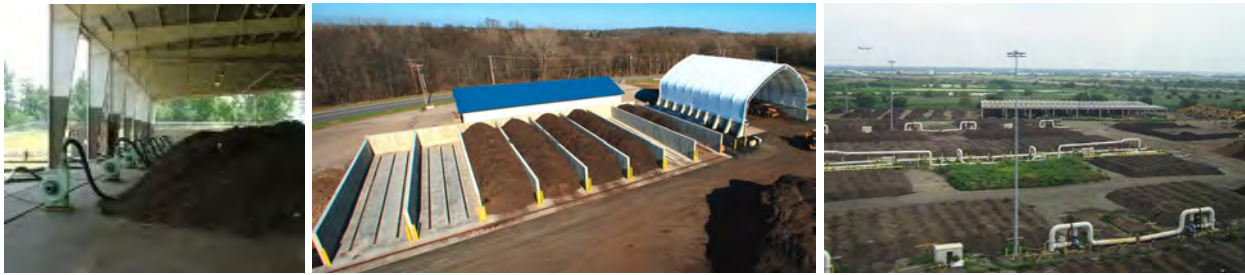
Figure 3-1. ASP alternatives in windrow (left), bunker (center), and extended ASP (right) configurations. Photos courtesy of Coker Composting and Consulting.
