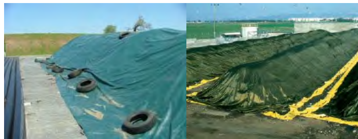
Figure 3-2. Fabric-covered ASPs. Photos courtesy of Coker Composting and Consulting.
