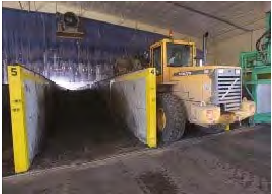
Photo 2 - Front End Loader “Charging” Bays
