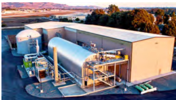
Figure 3-6. Horizontal Plug Flow Digester. Photo courtesy of BioCycle CONNECT LLC.
