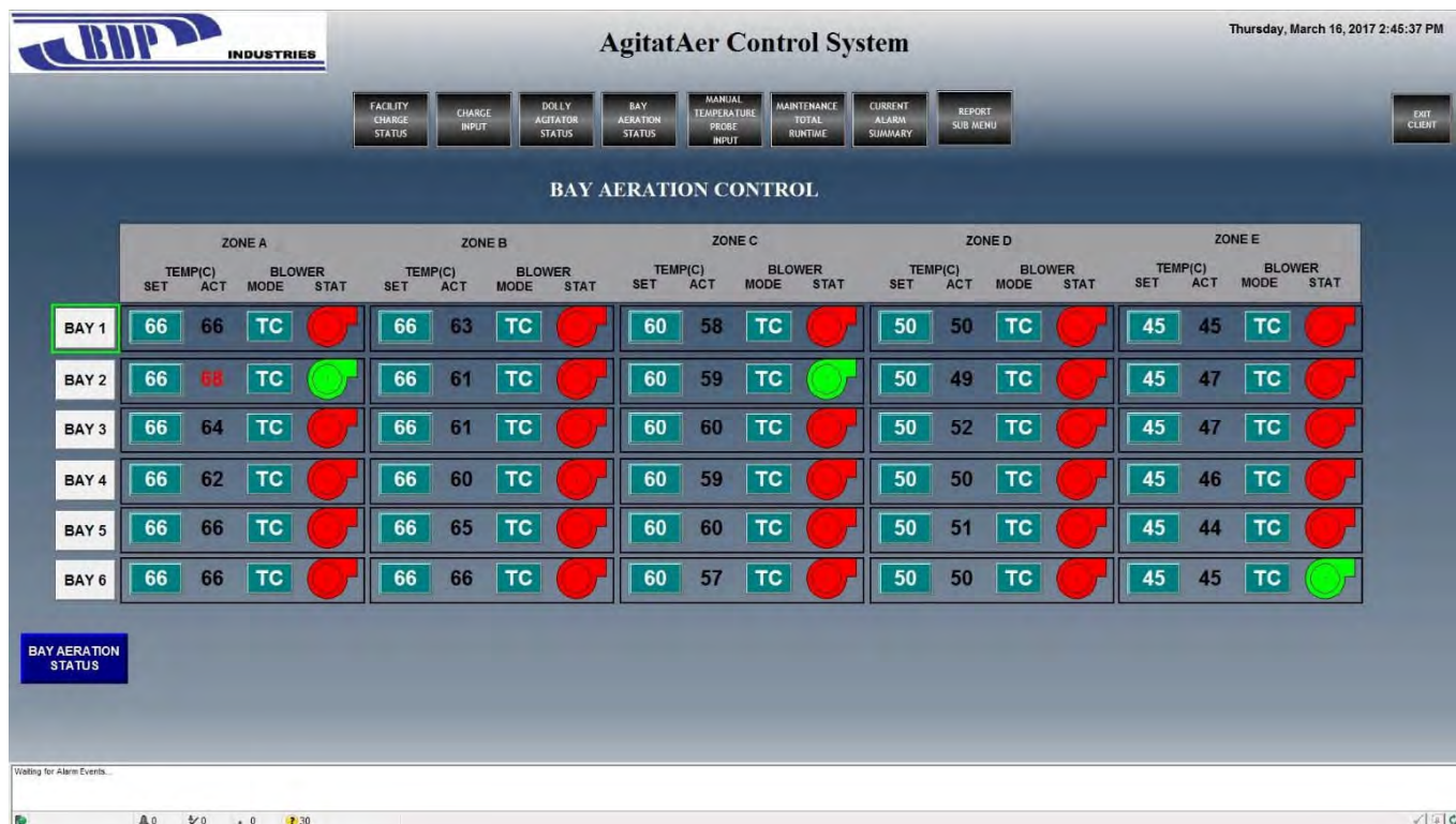
Photo 16 – Sample Blower Control Screen
