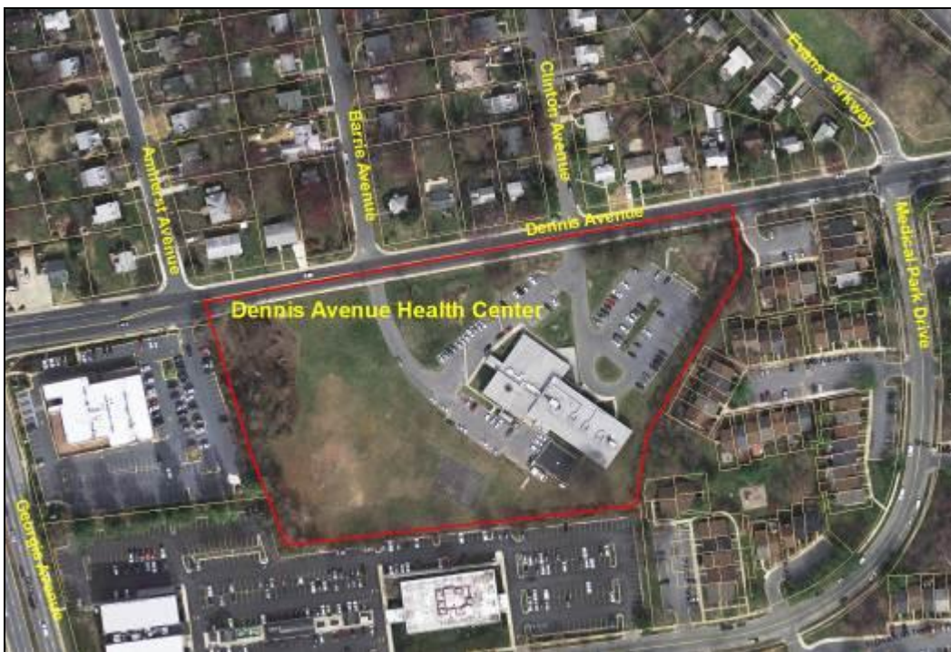
Figure 2: Existing Site Aerial
