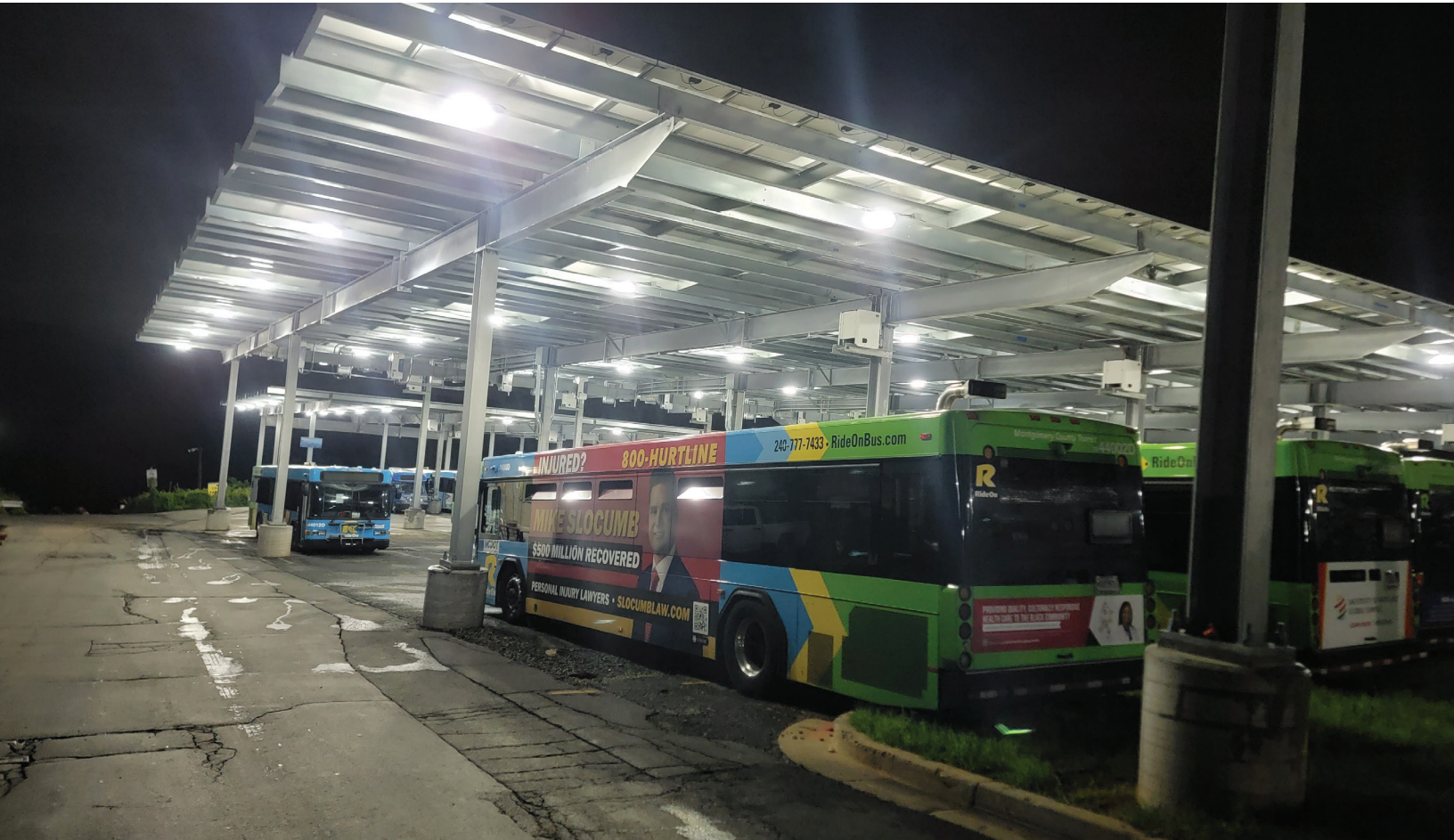
Brookville Smart Microgrid Solar Canopy and Bus Charging
